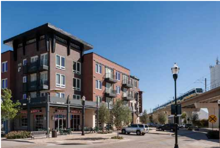
Apartments overlooking the DART transit line
